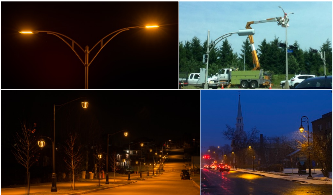
New PC-Amber LED luminaires installed inside the city of Sherbrooke. Multiple models of fixtures can be identified, from decorative to more regular streetlights.
