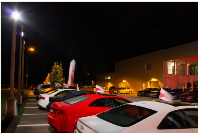
A pleasant surprise : a car dealership using Amber LED lighting! The front row of cars is lit with white LED for colour rendering while amber is used for the rest of the lot and the building entrances.
