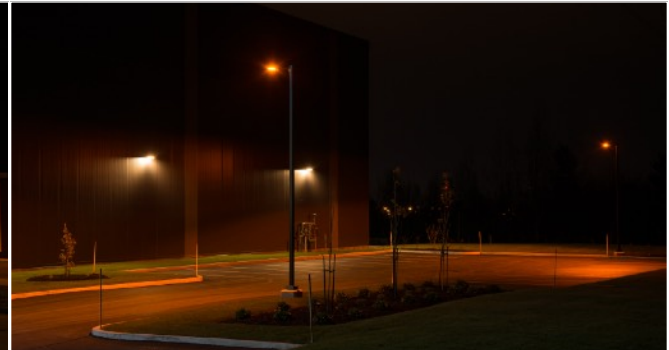
Monochromatic Amber LED and 2700K wall packs.
