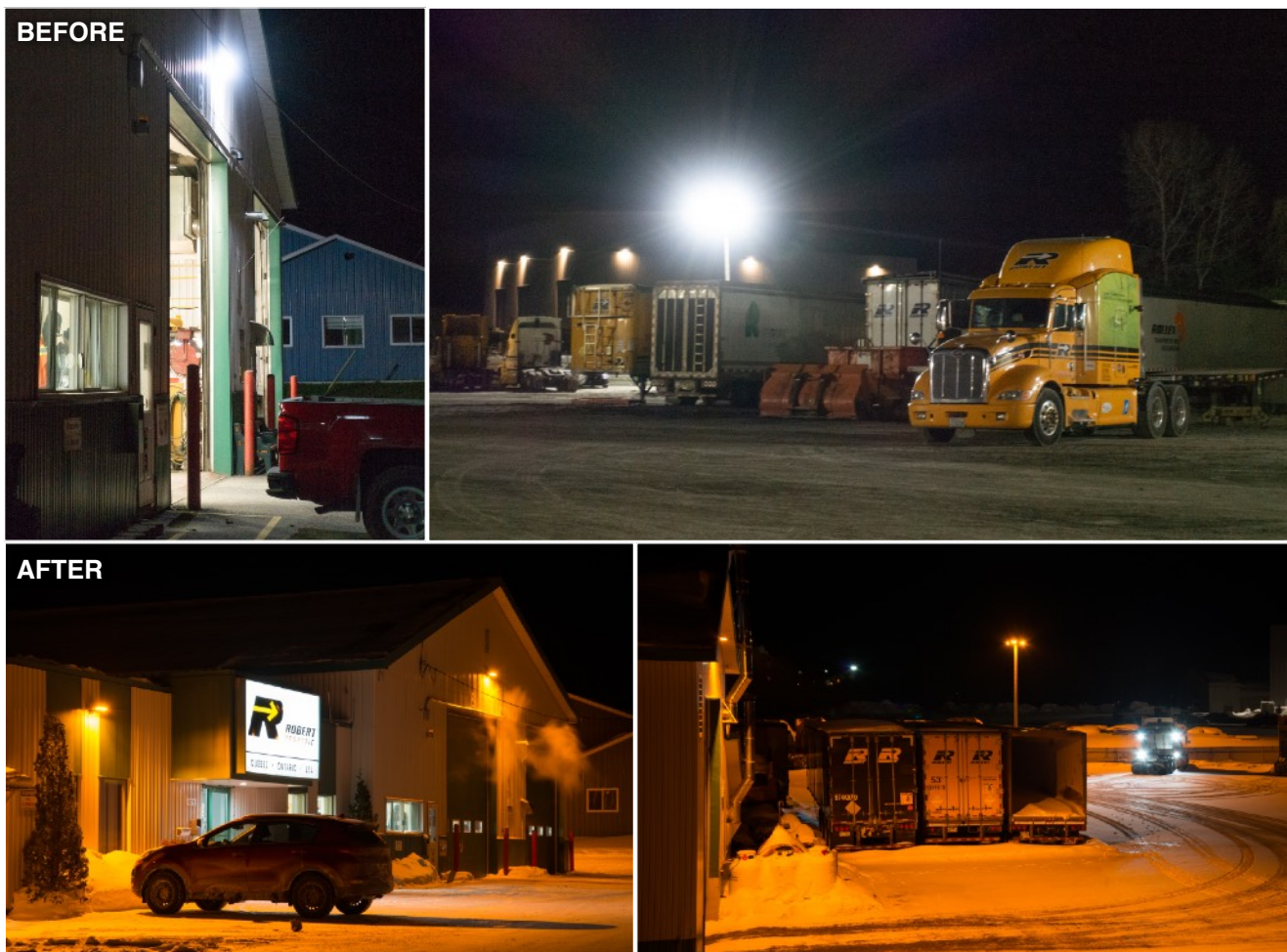
Before and after pictures of a transport company in Lac-Mégantic where cool-white LED were replaced with PC-Amber.
